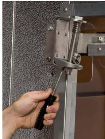
Hinge cam block adjusts with philips head screwdriver.
